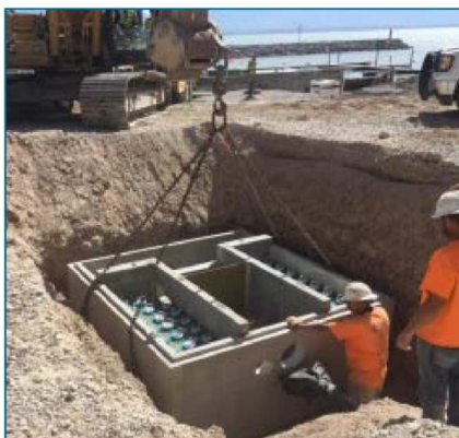
No deep sump chamber (as found with tentacle-type systems) and reduces excavation costs.
