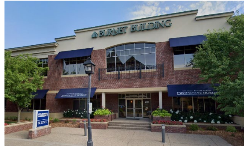
Stucco creates a lighter top but an odd transition
