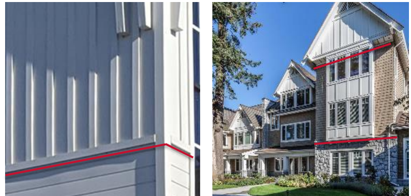
This material and trim may be wood or may be cement board siding.
