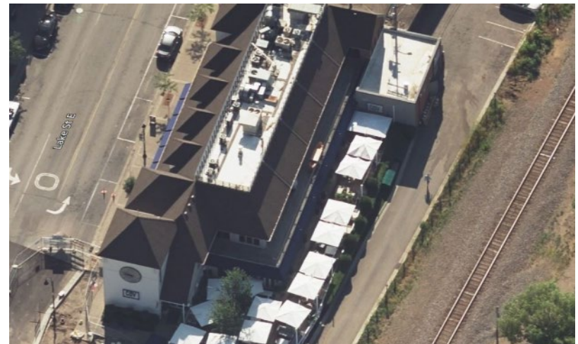
CoV uses sloped roofs at the visible perimeter while concealing a utilitarian flat roof from view.
