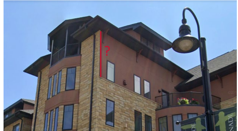
Material Change should be at the inside Corner for an appearance of solid material
