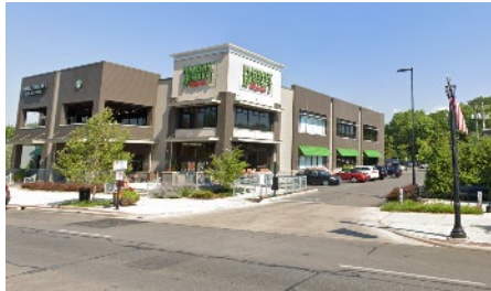
Single aisle side yard parking provides a compromise for this grocery store oriented perpendicular to the street.
