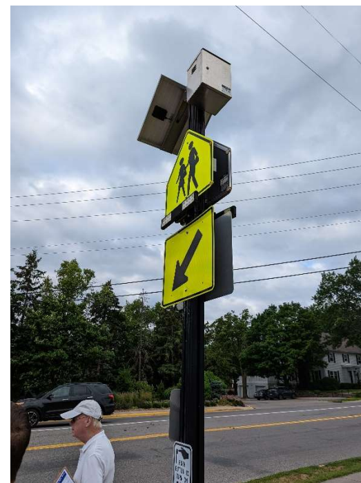
Existing Flashing Beacon at Barry Ave
