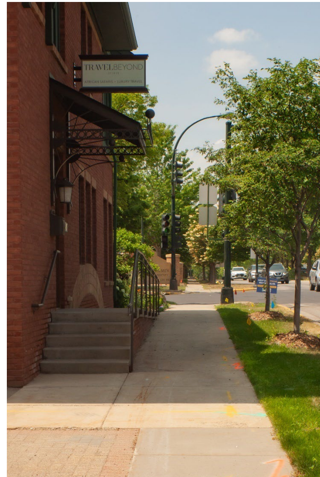
Existing Mixed-Use in the Town Core
