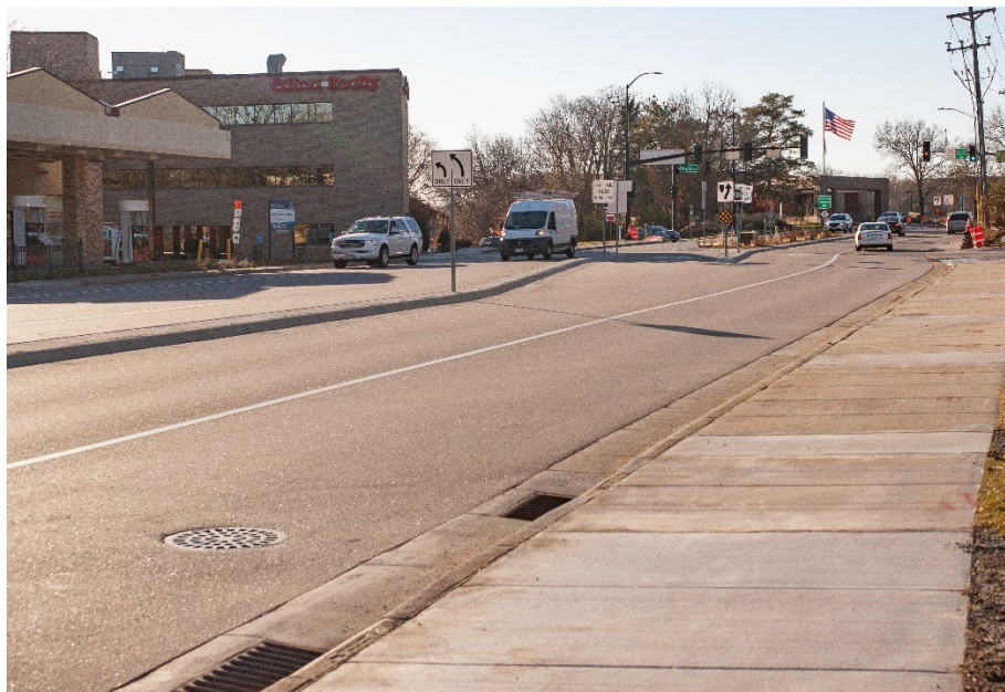
Wayzata Blvd at Central Ave looking west
