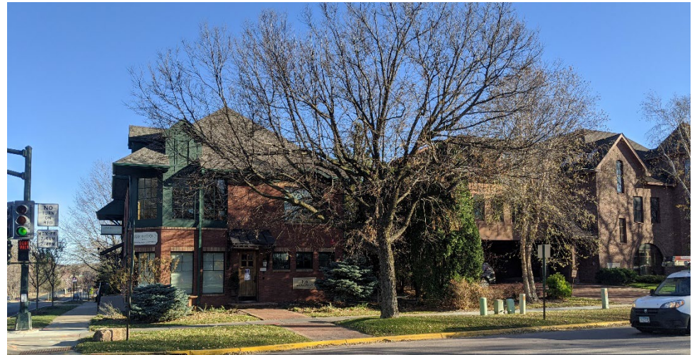
Existing Mixed Use in the Town Core
