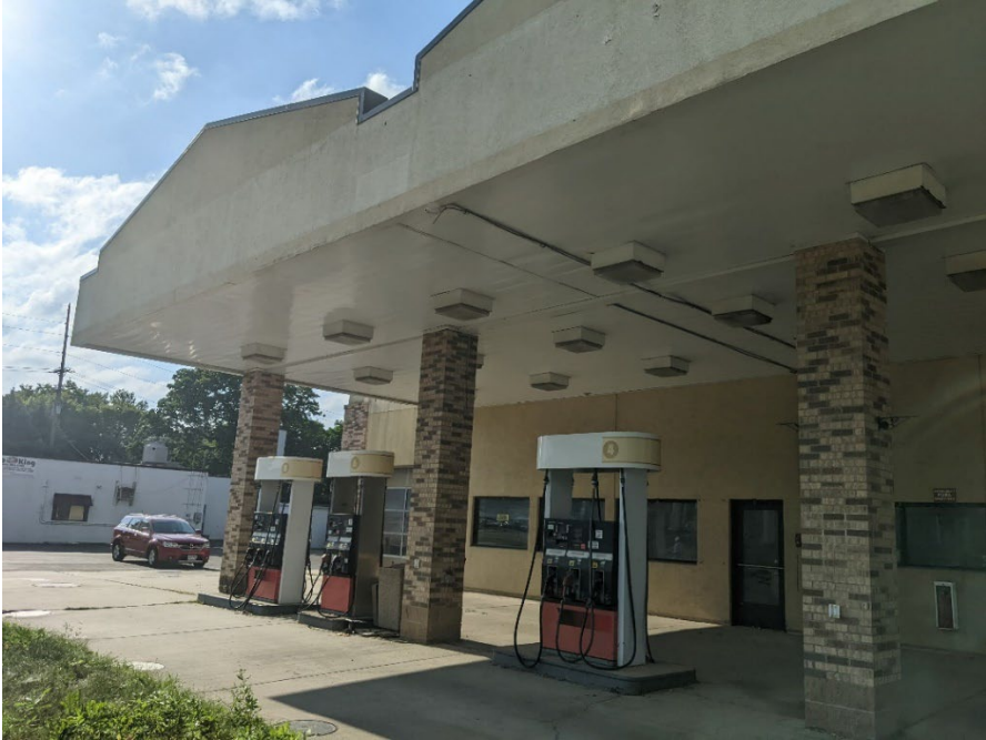
Former Gas Station
