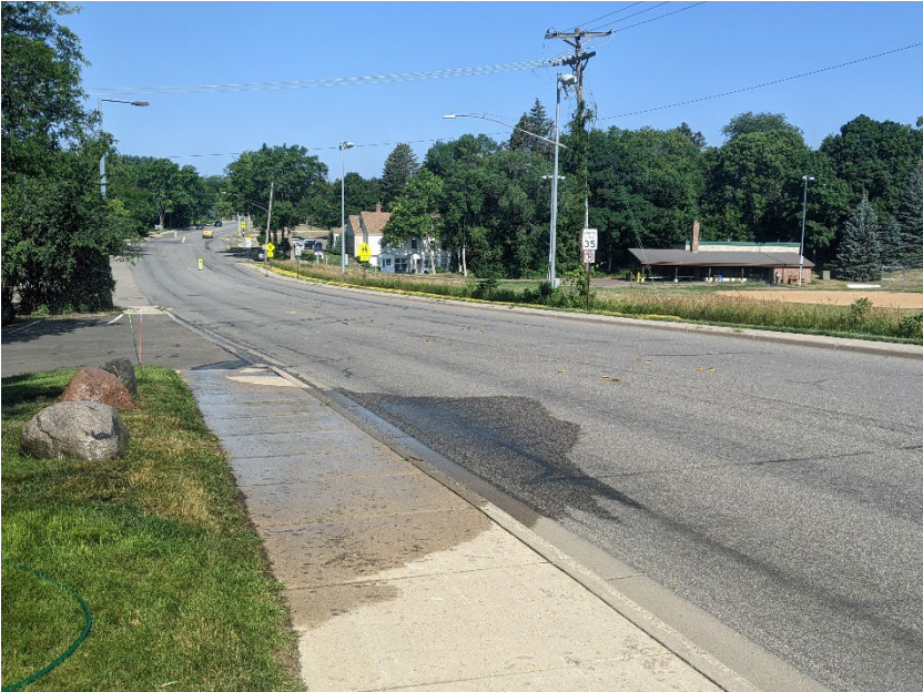
Wayzata Boulevard looking west toward Klapprich Park
